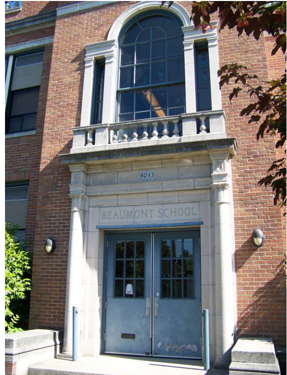
Main building (235A), looking north.
