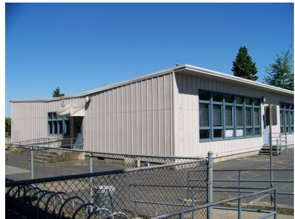
1948-1951 Portable Building (235A), looking northwest.
