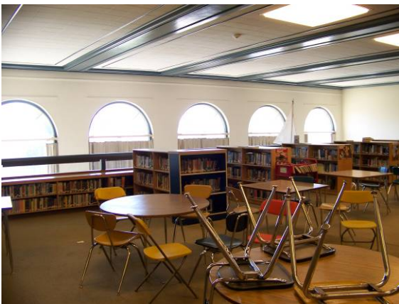
Main Building (235A), second floor media center (originally auditorium), looking southeast.
