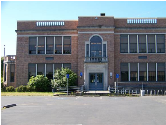
Main building (235A), looking south.
