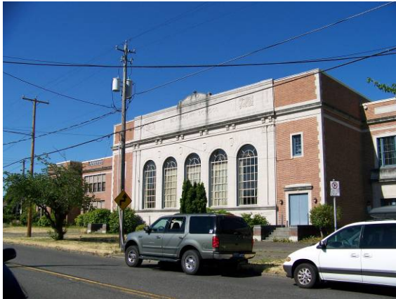
Main building (235A), looking southwest.
