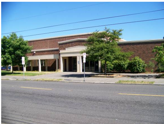
1989 Building (235C), looking north.
